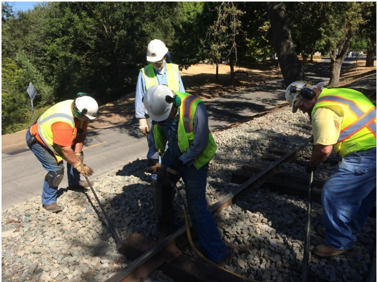
Frank and Mike F. "nip-up" the new tie as Steve drives the spikes with pneumatic spiker
