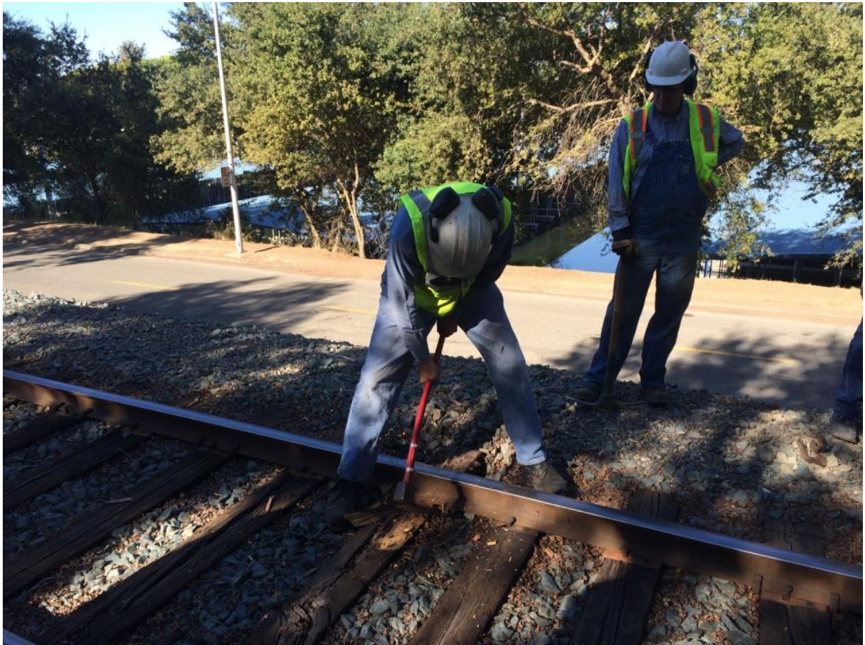
Alan uses the adz to chip away at a plate-cut tie in order to make it easier to slide out from under the rails
