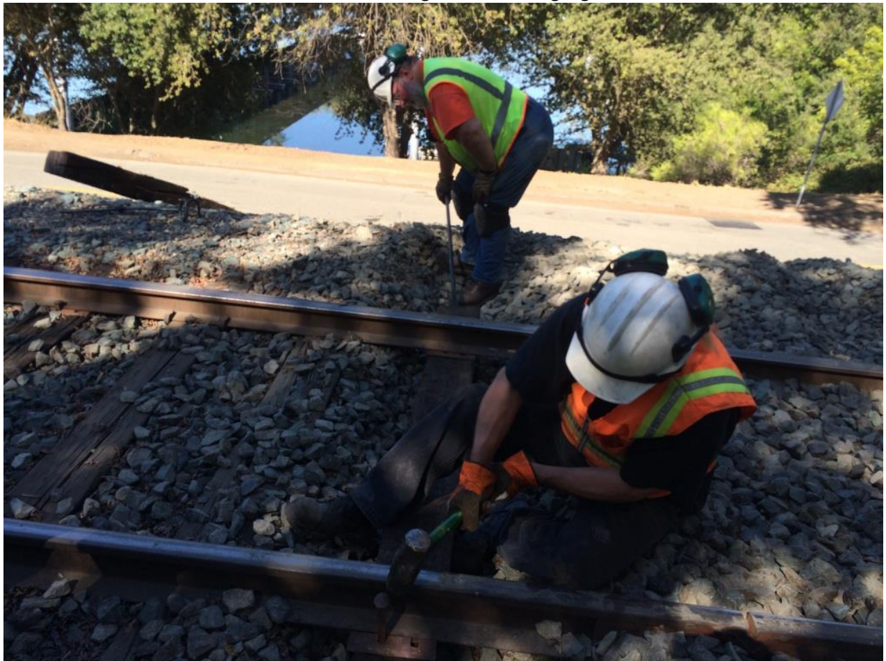
Frank "nips" the tie as Fred sets spikes
