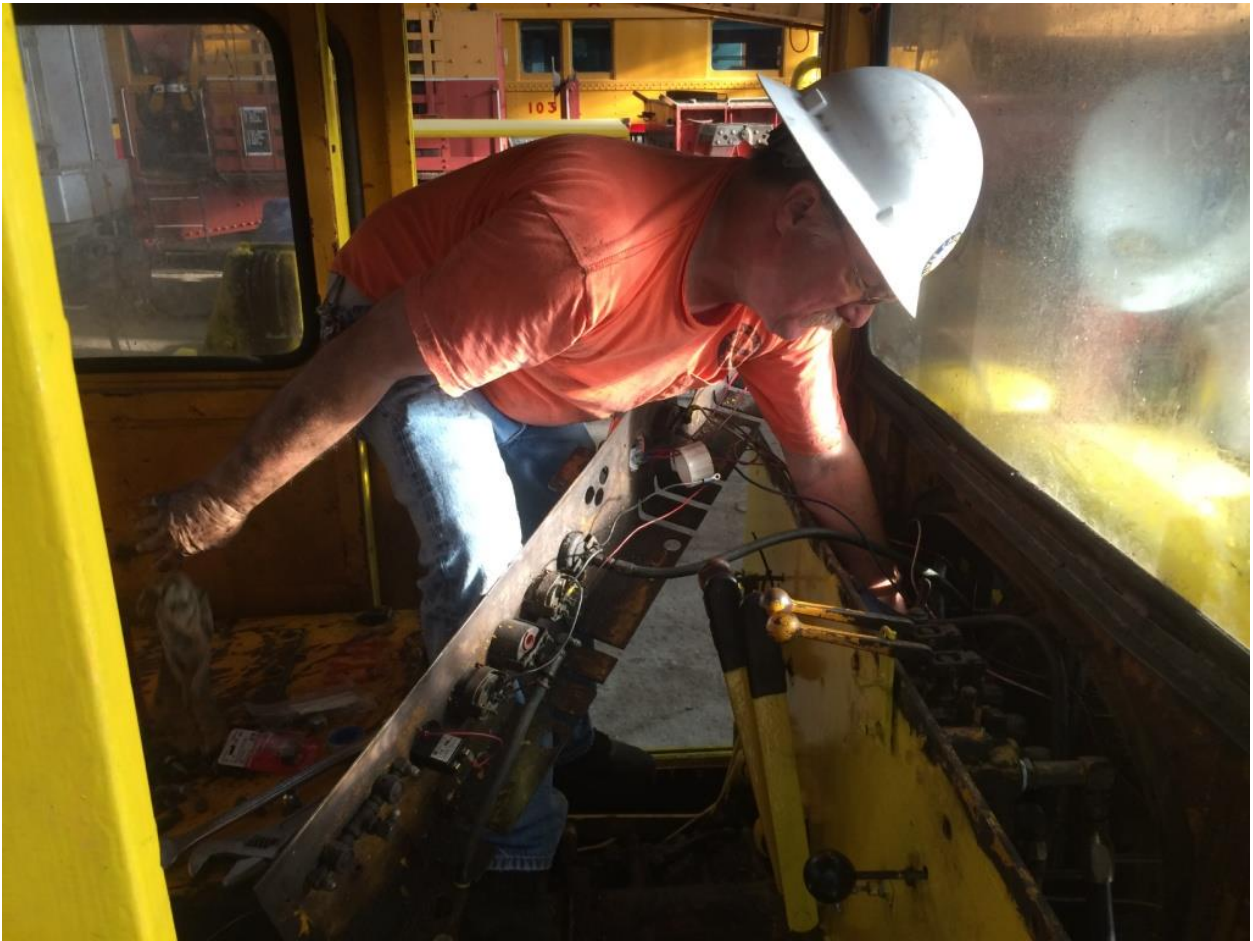
Mike H. deciphers the chaos that is the hydraulic plumbing of the Kalamazoo
