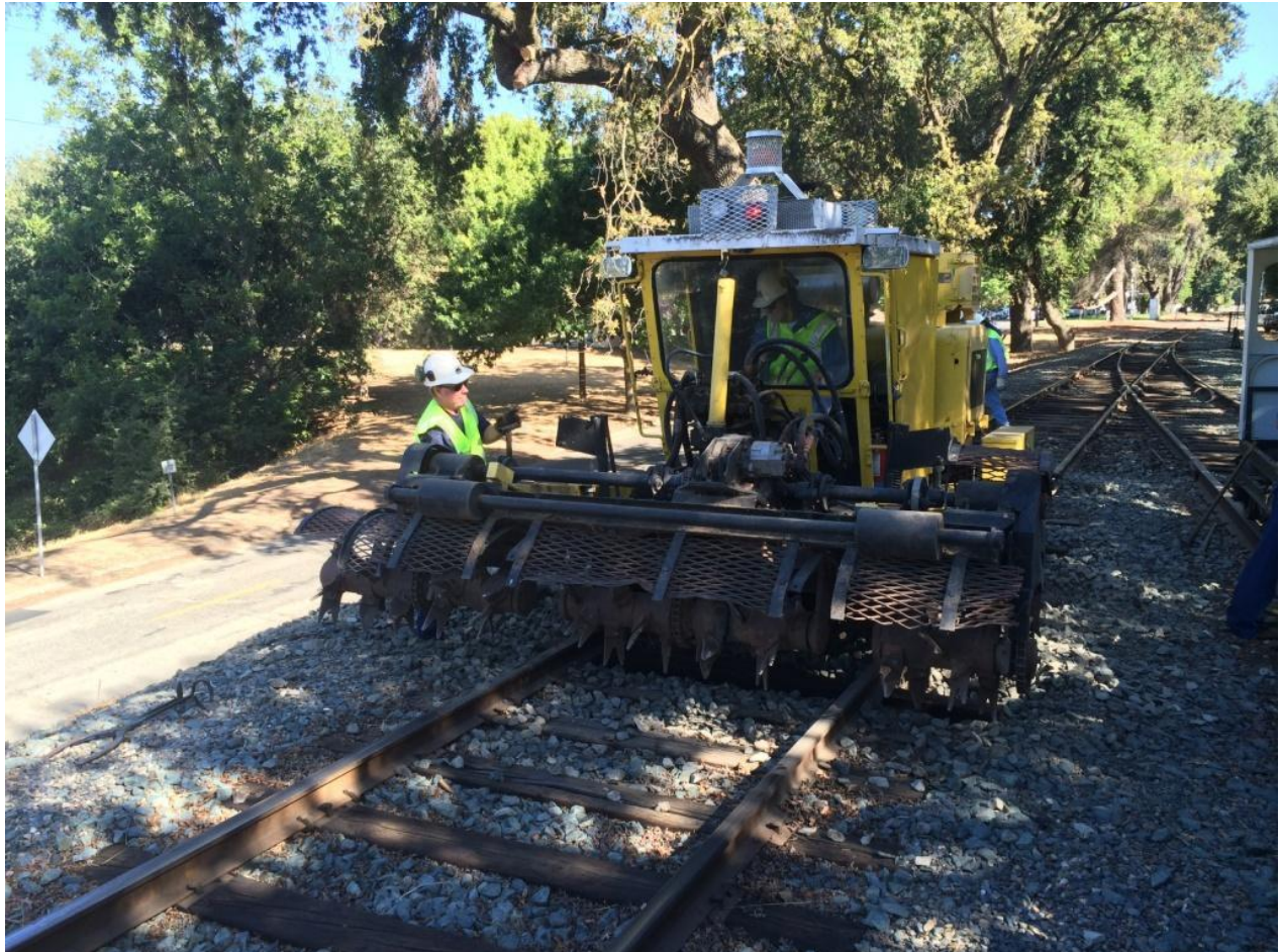
Ed guides the insertion of a new tie by the scarifer-inserter under Alan's capable hands
