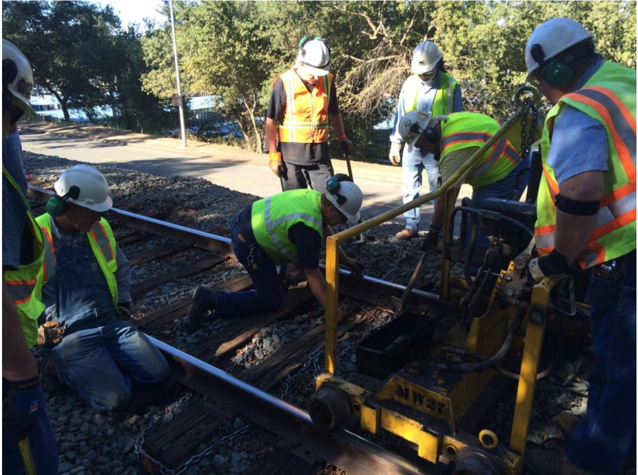
Steve, Ed, Fred, Mike M., Mike F., and Chris set up the section-gang machine's chains to remove a splintering tie
